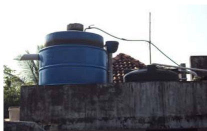
Figure 10: A 1m 3 domestic plant on the roof of a house in Kochi.
