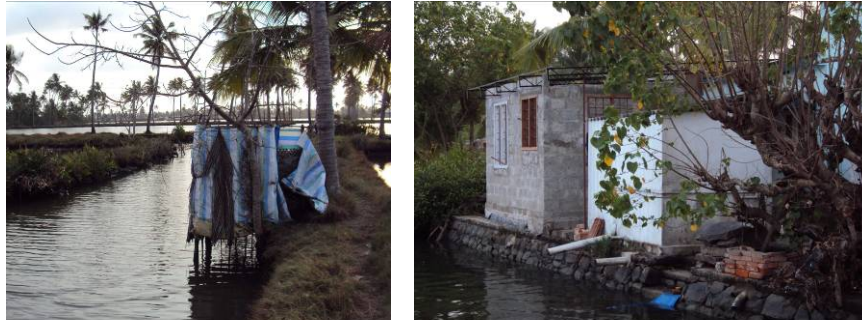
Figure 4: On the left (A): Hanging latrines (B) Latrines with an outlet discharging the human excreta into the backwaters.
