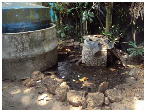
Figure 30: Accumulation of the effluent in the surroundings of the plant.
