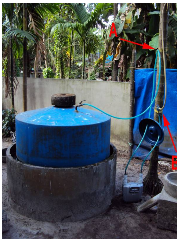
Figure 17: Connected gas meter. The fixation (A) enables the gasholder to move freely. The “three ways” installed at the point B enables to carry out \text{CO}_2 measurements.
