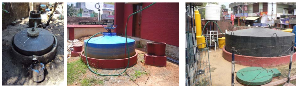
Figure 5: On the left (A): 1m 3 domestic plant. In the middle (B): 4m 3 institutional plant (HEEB, 2009). On the right (C): 4m 3 market plant equipped with generator (HEEB, 2009).
