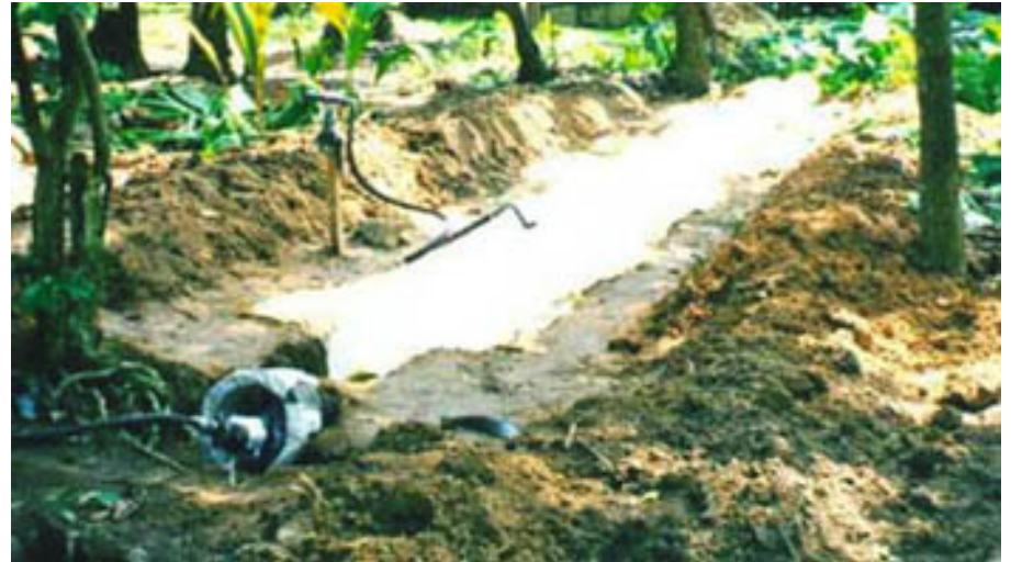
Figure 10. Photo of a biogas plant, filled with exhaust and water.
