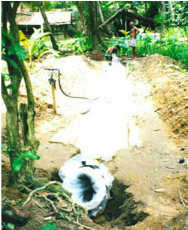
Figure 12. When water reaches the level of buckets, both ends are opened. Water level keep gases inside the bag, forming a bell.
