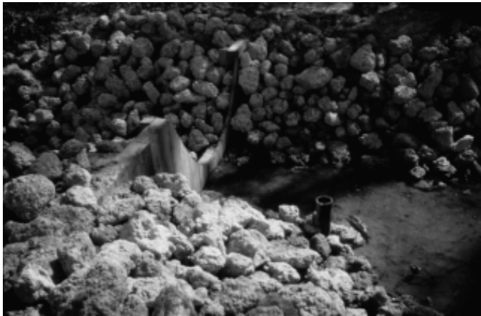
Figure 2. A typical retention device has two prominent features as shown in this photograph. First is the principal spillway. In this photograph the principal spillway is the wooden weir. The second is a draw-down device. In this case the small riser pipe has holes drilled into it behind the protective rocks. The difference in elevation between the drawdown device and the principal spillway dictates the wetland's temporary storage volume.
